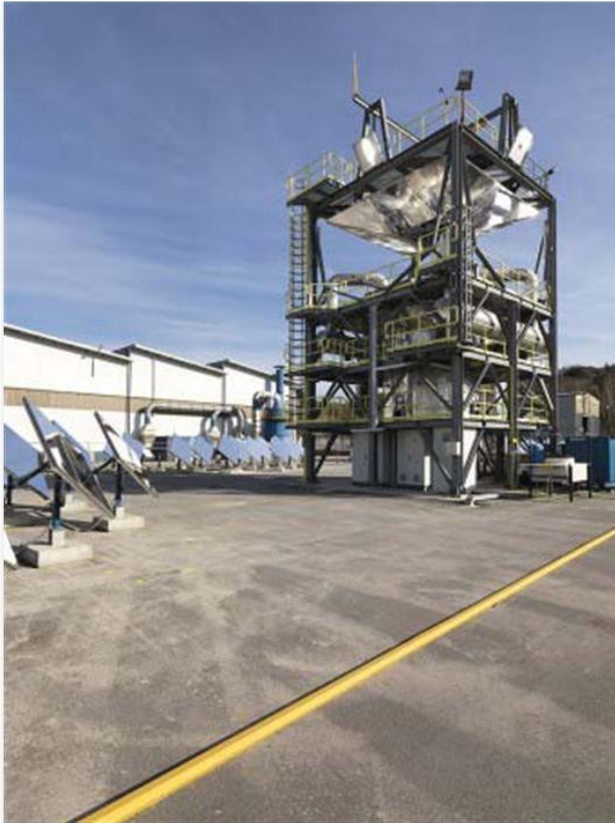
Stabilimento Magaldi _ Italy
