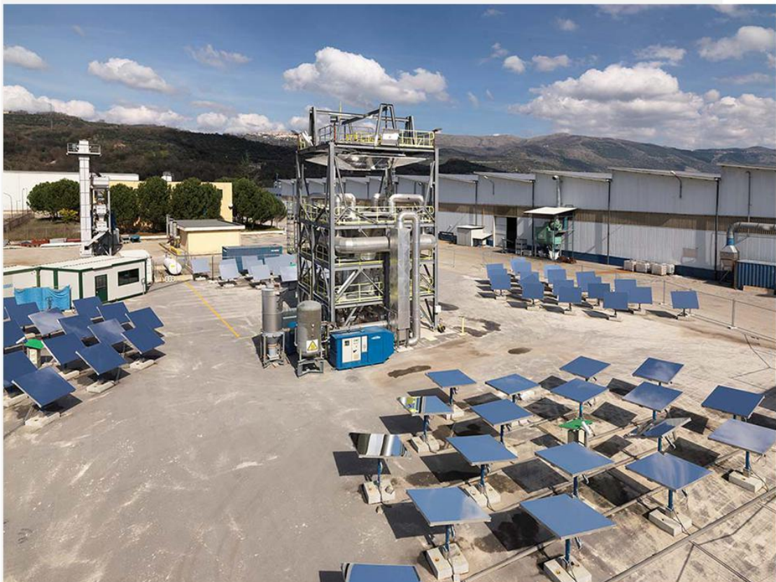
Stabilimento Magaldi _ Italy
