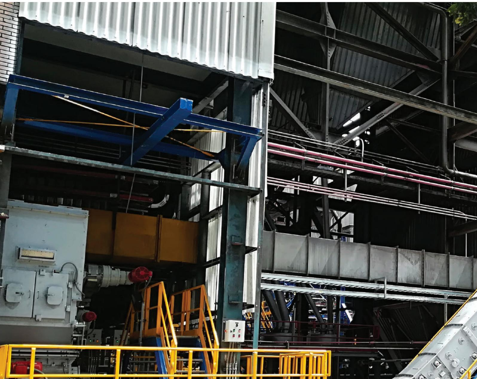
The MAC<sup>®</sup> (Magaldi Ash Cooler) is a unique system for dry extraction, air cooling and mechanical handling of bottom ash from pulverized coal-fired boilers.
